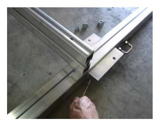
Loosen the angle brackets from the cross members enough to allow them to rotate.
