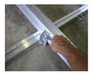
Attach the brackets to the tongue and tighten.
