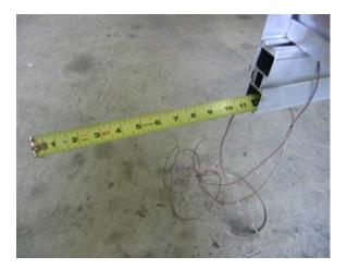
Extend a tape measure through the side rail and attach the brown wire to it.
