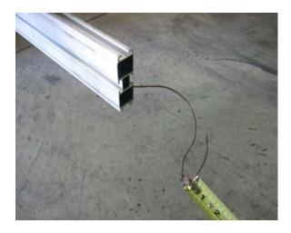
Retract the tape measure pulling the wire through the side rail until it comes out at the front.
