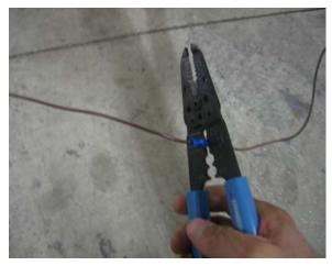
Install a butt connector by crimping it onto the bare wire.
